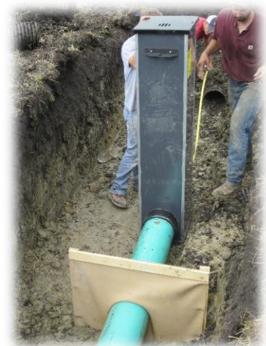
1. A drainage water management system structure being installed.
